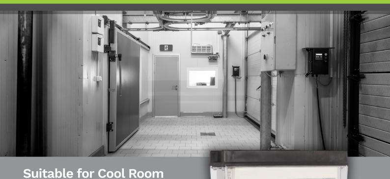
The Low Temperature Exit range is designed for cool room and freezer applications where the temperature can drop to -40°C. The range consists of IP66/67 exits that include lithium battery technology which ensures significant maintenance savings compared to other alternatives.
